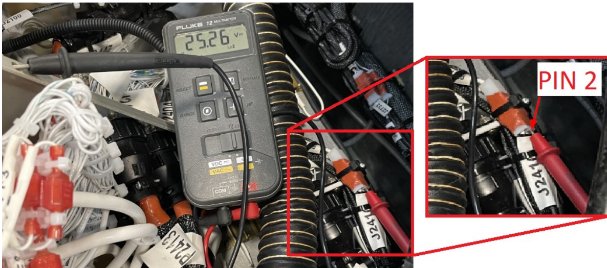
Figure 2. Voltage check of pin 2.
