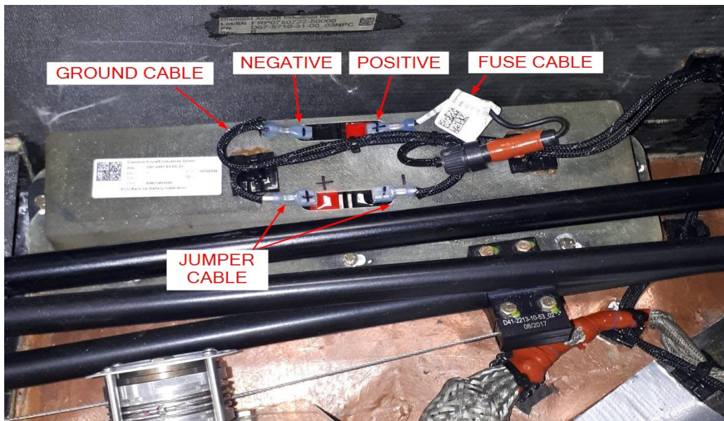
Figure 5. RH battery (cables connected).
