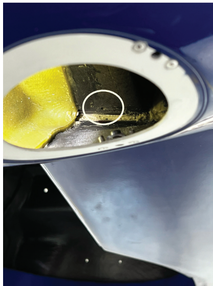
Drain Holes (Locations 3 & 4)
