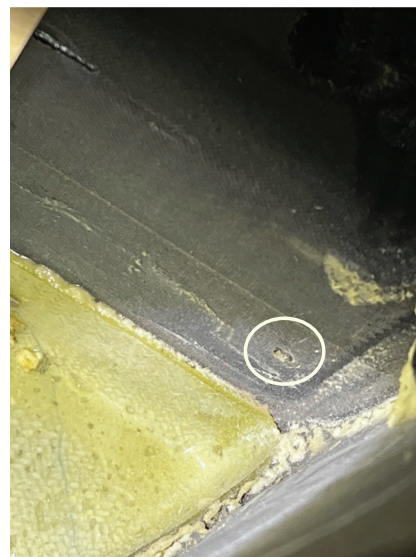
Drain Holes (Locations 9 & 10)
