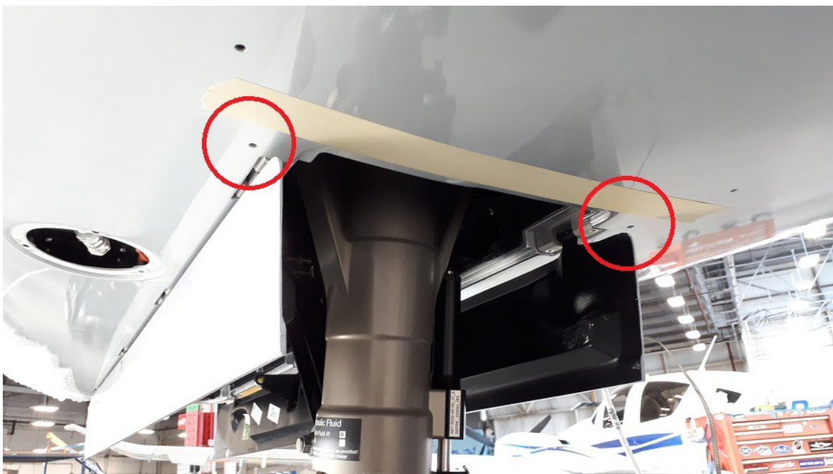
Figure 1. Drain holes to be drilled under the LH nose baggage compartment and the avionics bay.
