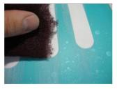
10 Clean the surface of Safety Walk cutouts with vacuum and silicone remover.
