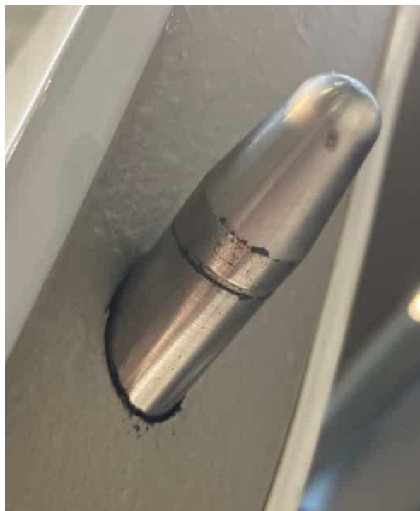
Figure 14. Example of serviceable latching bolt
