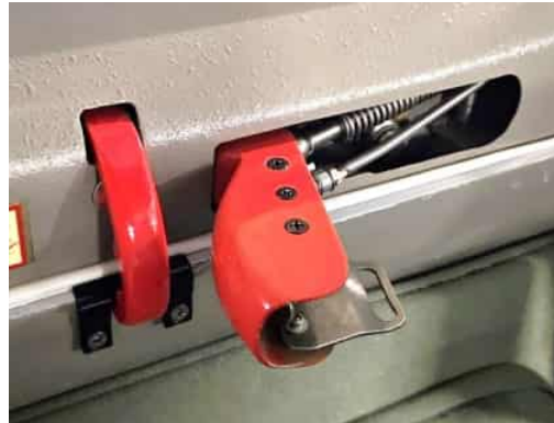
Figure 8. Old door latching mechanism
