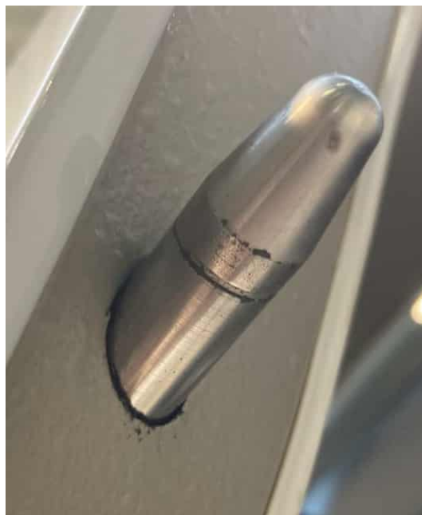
Figure 14. Example of serviceable latching bolt
